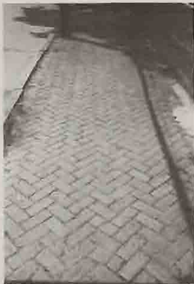
Herringbone brickwork in sidewalk on Kirkland.
