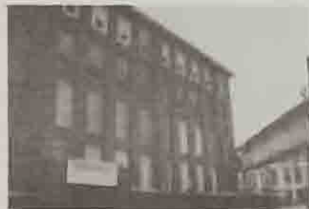
Top: Windows on west side of Fulton Mill.
